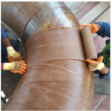
A two person crew was sufficient to apply the Wax-Tape® HT-3000 wrap on the 24" pipe bend.
