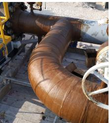
In tight quarters, the advantage of the Trenton Wax-Tape® wrap system over other solutions is the ease of surface preparation and application as compared to an abrasive blasting or a bulky wrapping machine.
