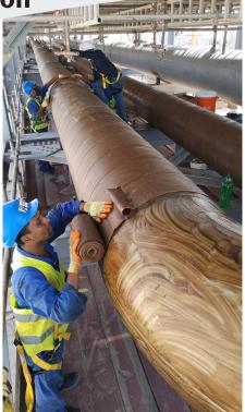
The spiral wrapping of Wax-Tape<sup>®</sup> HT-3000 wrap on a 30" pipeline proceeds quickly.
