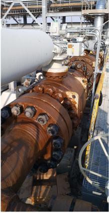
Temcoat<sup>™</sup> 3000 and Wax-Tape<sup>®</sup> HT-3000 wrap provided protection of a motorized valve and flange on a 10" pipe.
