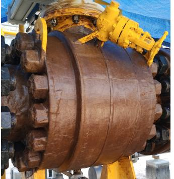
was coated with the Temcoat<sup>™</sup> 3000 primer and Wax-Tape<sup>®</sup> HT-3000 wrap system. The conformability of the wrap meant that it could be applied without a mastic, making the application process fast and enabling a rapid inspection.
