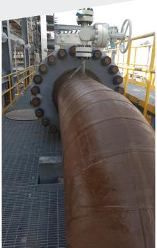
A 30" pipeline protected with Temcoat<sup>™</sup> 3000 and Wax-Tape<sup>®</sup> HT-3000 wrap before the insulation was applied.
